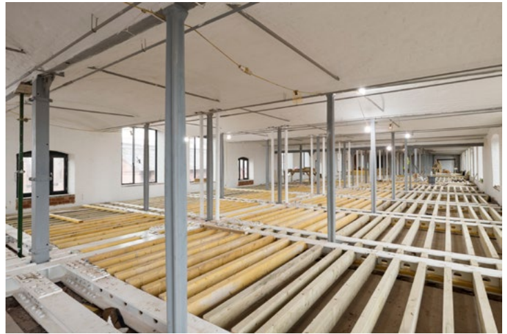
©Steve Baker, Historic England – first floor Main Mill with new additions – new steel grillage to floor; tie rods at the ceiling and reopened flax era windows, September 2020
